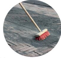
In this system, you need to use right particles sizes are used of top of each layer in order to achieve the desired result. It is designed to provide a strong, durable and permanently water-permeable joint filler according to current regulations and recommendations by the Belgian Road Research Centre.
