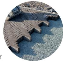
It is recommended for H<sub>2</sub>O bedding course with a fraction 2/4 or a split with a fraction of 2/6.2 to be used for the laying bed. It is preferable not to use the fraction 2/8 in order to avoid the risk of the joint split being washed away.
