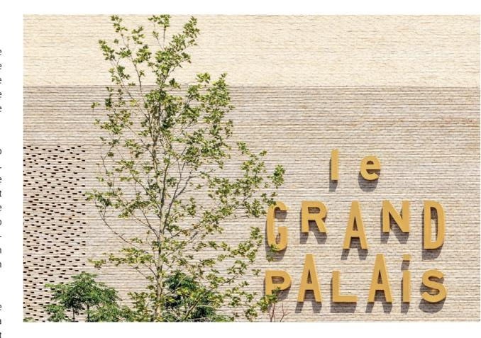
This alternation between open and solid parts of the façade is based on a functional logic. The perforated envelope enlivens the internal spaces during the day and creates an intriguing interplay of light and shadow at night, with tiny shimmering lights creating a magical effect when viewed from outside.
