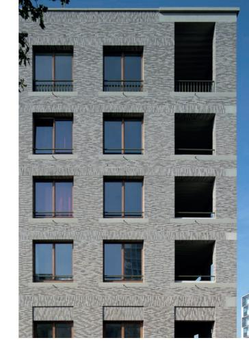
Hama combined these two Linea facing bricks with a transparent green glazed brick which has also been used in the communal entrance halls and interior spaces. Like the facing bricks, the glazed bricks also have a Wasserstrich texture which is still clearly visible through the transparent glaze. This creates an extremely lively surface in terms of the glazing and colour variation.
